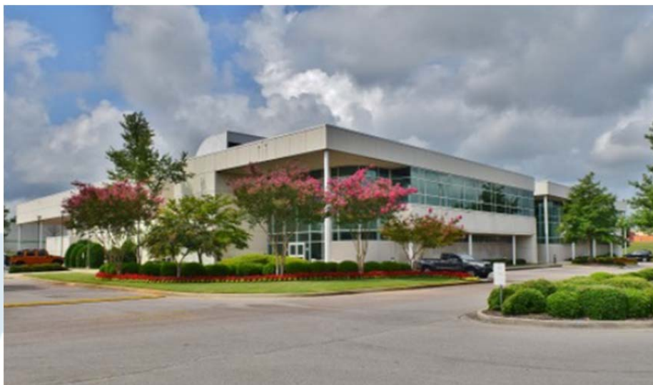
The new EOS facility in Huntsville, Alabama.
