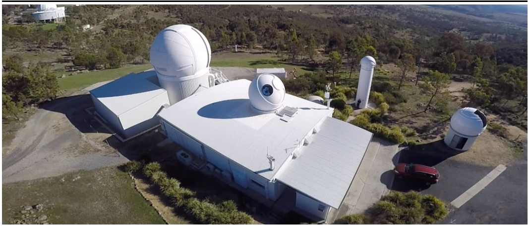
Figure 4: EOS Space System Laser Site
